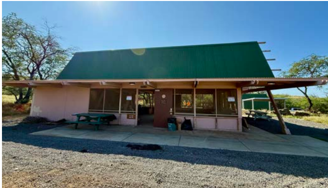
Pavilion at Hapuna State Recreation Area
